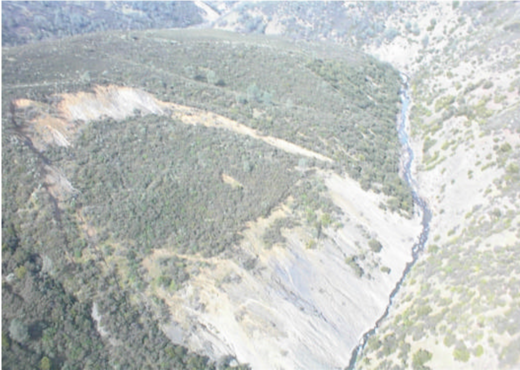
Photo 1. North Fork Cache Creek Landslide (2001)
